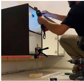
Install kitchen, cabinets and HVAC equipment. Installation de cuisines, armoires et appareils CVC.
