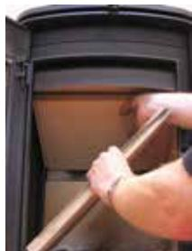
3. Tilt one of the side brick panels and remove it.
