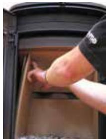
2. Tilt one of the side brick panels and remove it.
