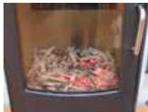
6. Place 2 pieces of wood of approx. 0.7 kg each and approx. 25-30 cm long over the embers in a single layer, with a distance of approx. 1 cm.
