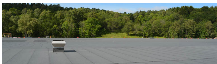
Figure 1. Example picture of installed Icopal Mono reinforced bitumen sheets.
