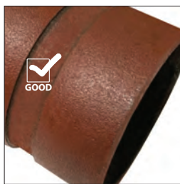
GOOD PIPE END DOES NOT CONTAIN ANY DAMAGED PAINT ON THE "A" DIMENSION
