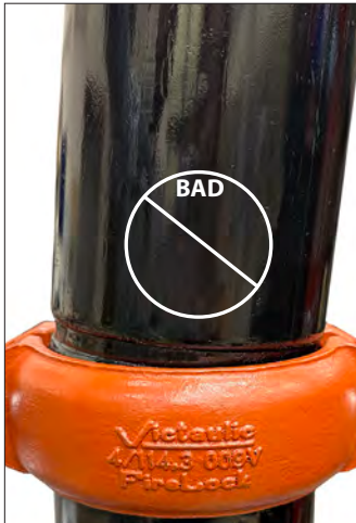
PHOTO 1 (UNACCEPTABLE) – EXCESSIVE INSERTION ANGLE
