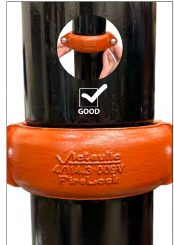
PHOTO 4 (ACCEPTABLE) – HOUSINGS' KEYS ALIGNED WITH PIPE GROOVES
