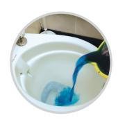
2. Pour the mix into the waste system which needs tracing.
