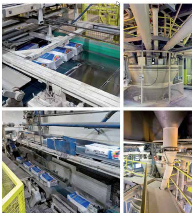
Figure 1: Production process detail
