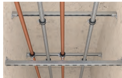
Pipe fixing in a corridor
