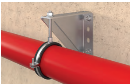
Heavy drainage pipe under angle bracket
