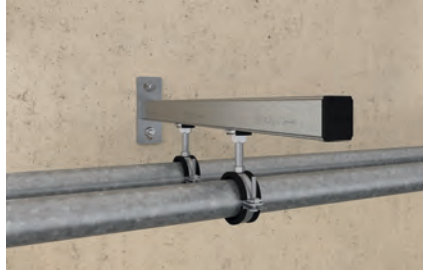
Light pipe fixing
