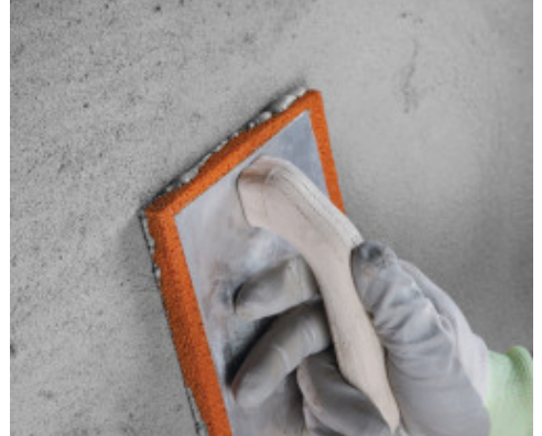
Tamping Planitop Smooth & Repair Zero
