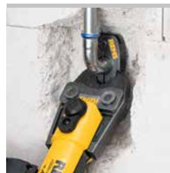
REMS pressring 45° (PR-2B) Patent EP 2 774 725
