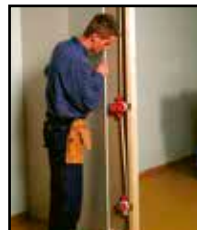
Monter gipsplate /panel.
