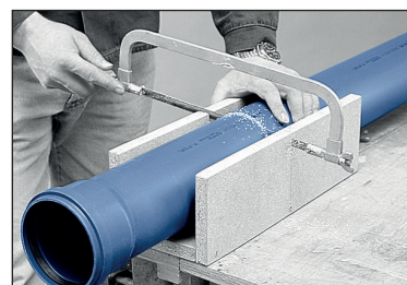
Cutting to length with a fine-toothed saw (FIGURE 20)
