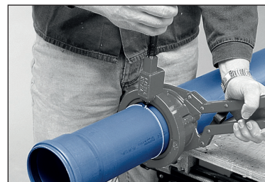
Cutting to length with a cutting and chamfering tool (FIGURE 19)
