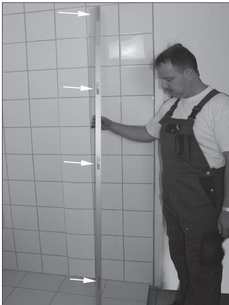
Space out the four wall plates along the profile, place them in the screw holes and secure them loosely with the nuts. Follow the gluing process for application of glue and cleaning.
