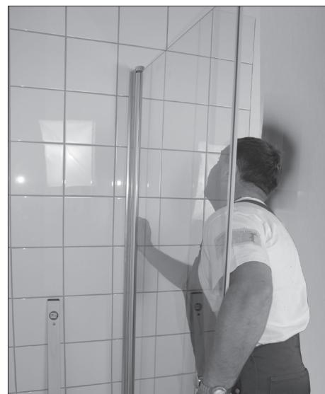
Then install the glass in the wall profile, adjusting and fixing the glass in accordance with the shower partition instructions. **DONE!**
