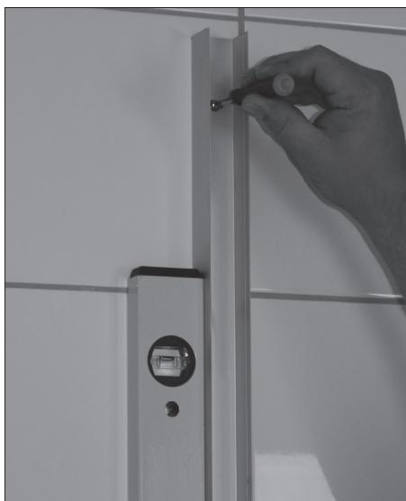
Leave the glued plates to harden for 24 hours at normal room temperature. Then mount the profile on the wall plates again and lock in place with the nuts. **Tip!** Use a 7 mm socket spanner for easy access to the profile and to lock the nuts in the plates.
