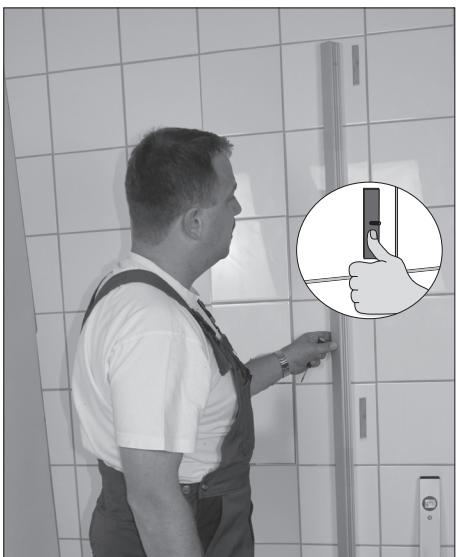
Loosen the nuts and carefully remove the profile from the wall. It is important to check that the wall plates are attached to the wall. Press them hard! Check that the hole spacing in the profile matches the position of the plates. Adjust as necessary.
