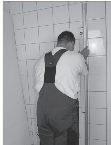
Measure the space for installation in accordance with the shower partition instructions. Then press the profile firmly against the wall and check that the profile is straight and plumb.
