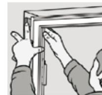
**EN:** Wedge the sides of the frame at the top with temporary double wedges. Check with a long spirit level that the frame sides are plumb and square.
