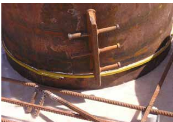
Overgang stål / betong
