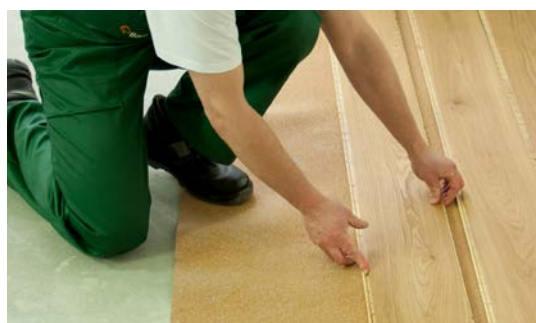
Fig. 3. The view of 3-layer wooden floorboard produced by Barlinek Inwestycje Sp. z o.o. during installation
