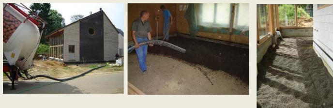
Figure 4: Blowing with manual levelling installation
