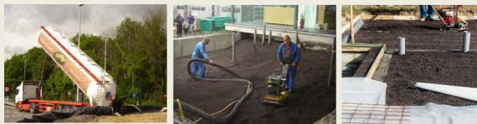
Figure 3: Blowing with vibrating plate levelling-compaction installation
