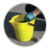
**1.** Mix drain dye with water. 1 teaspoon of drain dye to approx 10 litres of clean water.
