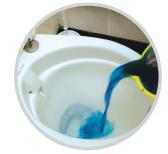
**2.** Pour the mix into the waste system which needs tracing.
