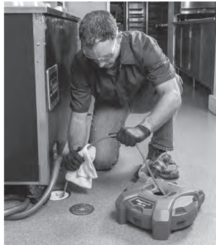
Figure 15 – Applying Lubricant to the Cable Sheath
