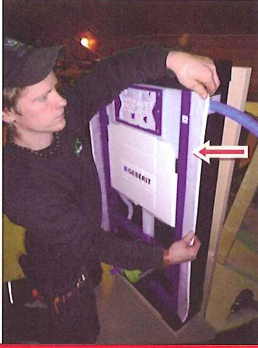
A photograph showing a person wearing a dark cap and jacket, applying a purple seal strip to the edge of a white wall panel. A red arrow points to the seal strip being applied to the top corner of the panel. |
